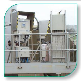
Designed to operate under legislation such as 2000/76/ EC (WID) and 2001/80/EC (LCPD), The MIR-IS offers maximum availability and complete compliance with QAL 1 of EN14181 & EN15267-3.
