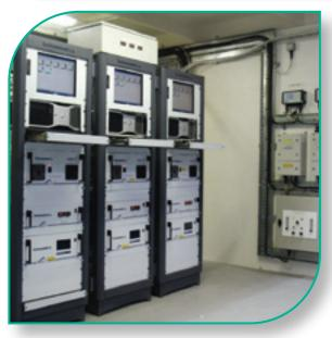
The MIR-FT is rack mounted in air conditioned enclosures. Complete systems would normally comprise of:
