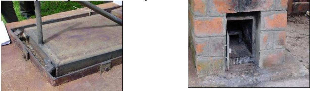
Figure 3 Photos indicating maintenance problems for De Montfort Incinerators in Kenya. All from Taylor (2003). Left: Front door hinges damaged and frame dislodged from mortar. Right: Damaged masonry and loose fire-bricks
