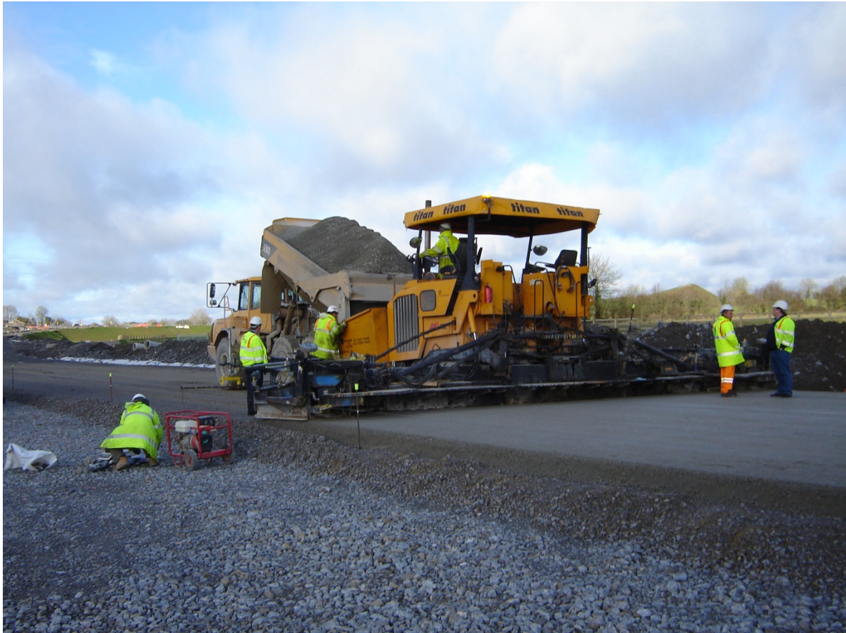
Use of Incinerator Bottom Ash Aggregate. Image courtesy of Ballast Phoenix
