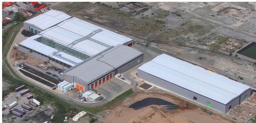
Avonmouth MBT / ATT facility. Image courtesy of New Earth Solutions.
