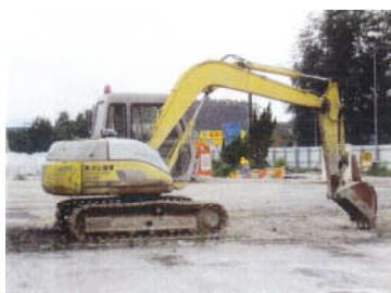
Excavator at construction site
