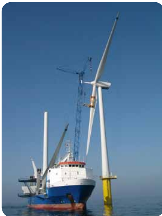
Offshore wind turbine installation.
