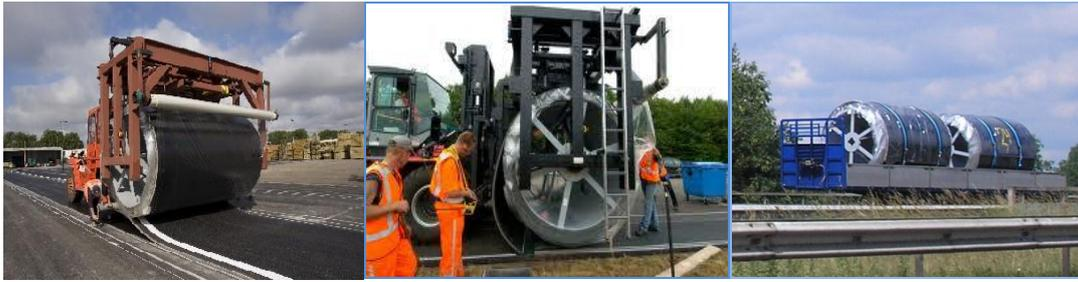
Rollpave has been tested and under observation on a couple of bypasses of highways in Netherlands under a test called “Road to the Future” program sponsored by the Dutch Road Authority.
